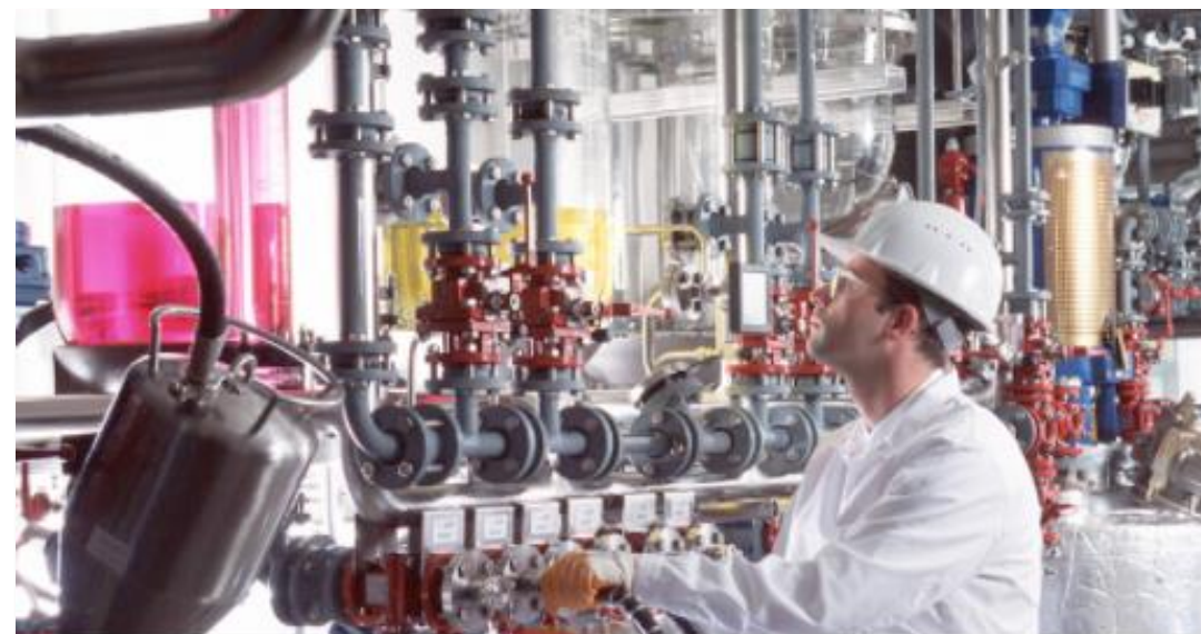
LANXESS enters battery chemistry business: electrolyte production for lithium-ion batteries in Leverkusen, Germany
